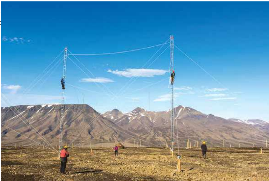
Figure 12: The SuperDARN radar under construction
